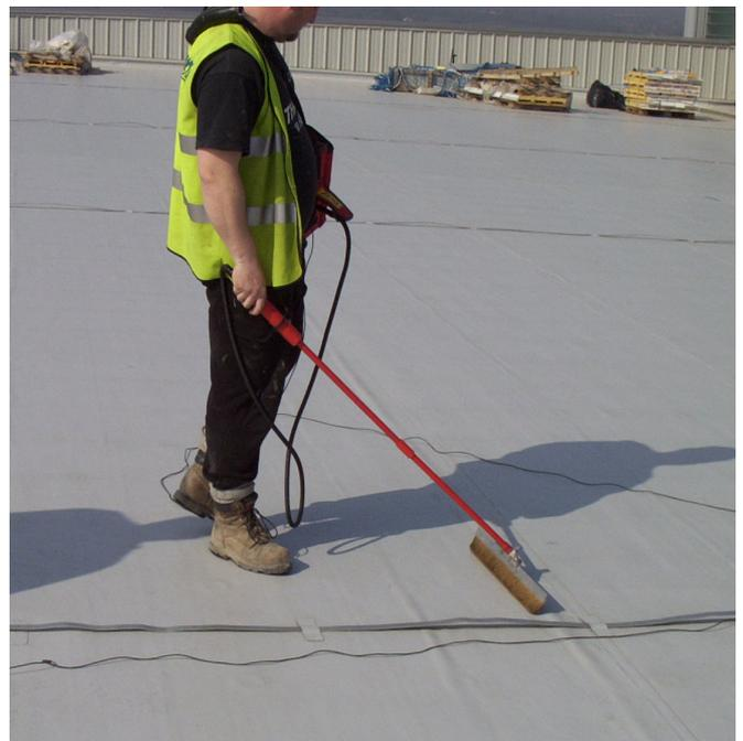
Testing should be continued across the complete surface and all faults marked. Damaged areas should be re-tested after repairs have been carried out.
